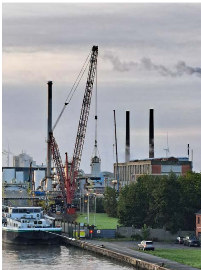
Picture: Install drying tower during sulphuric acid shutdown
